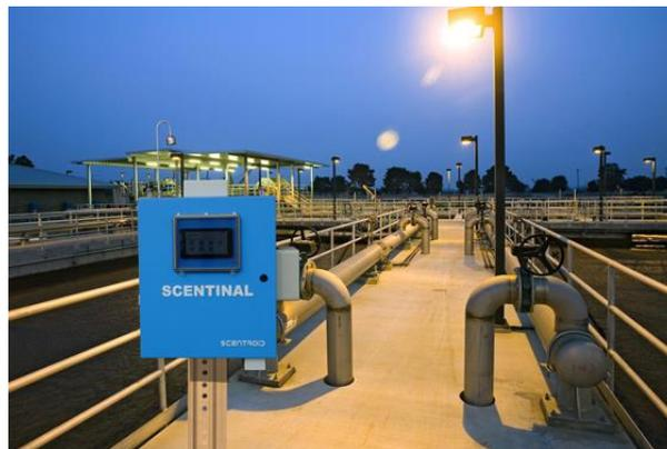
Scentinal provides ambient odor emission monitoring based on high accuracy (ppb level) detection of odorous gases such as H<sub>2</sub>S, Ammonia, VOCs, and SO<sub>2</sub>. The flexible intelligent station allows live monitoring of plant emissions on Scentroid's cloud servers. Odor emission is reported in OU/m<sup>3</sup> based on correlation determined based on periodic measurements using field olfactometry.
