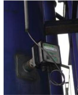
Electrodynamic Sensor installed in bag house outlet
