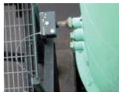
Pro-Scatter and Electrodynamic Main Stack Sensors
